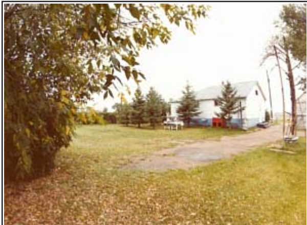
Looking at the back of the grocery store purchased by the church for renovation.
