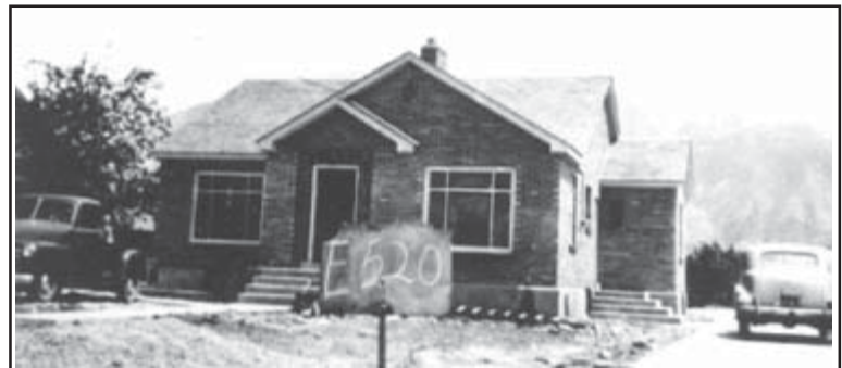
We lived in the basement until the upstairs was completed.
